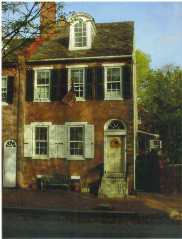
Figure 6-4 New James McCullough House.
