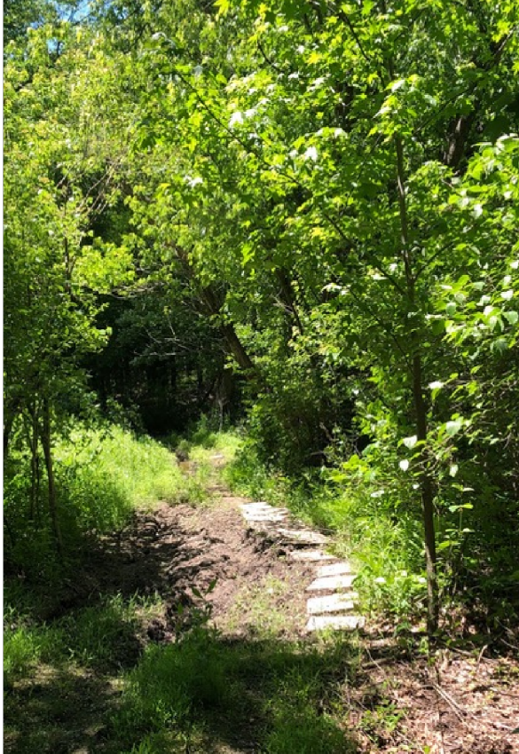
Before and after vandals sawed and removed the plank bridge.
