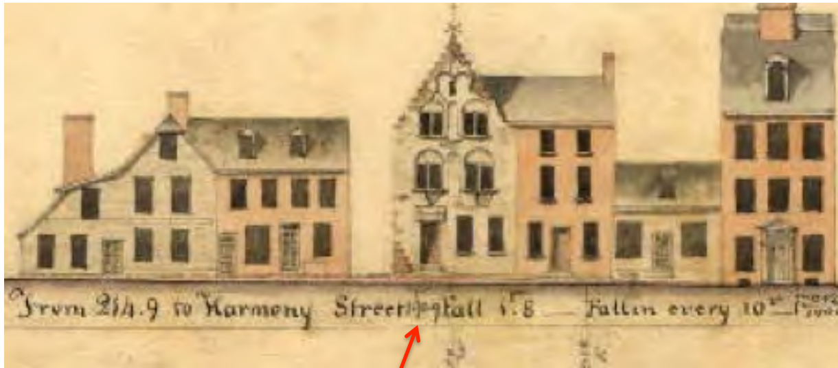
Thomas' Hotel, now Episcopal Parish House
