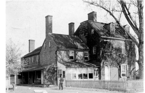
Built east half The Hermitage
