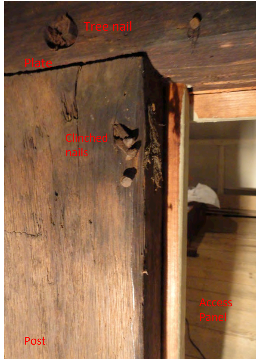
Closeup of top of plate and top of post
