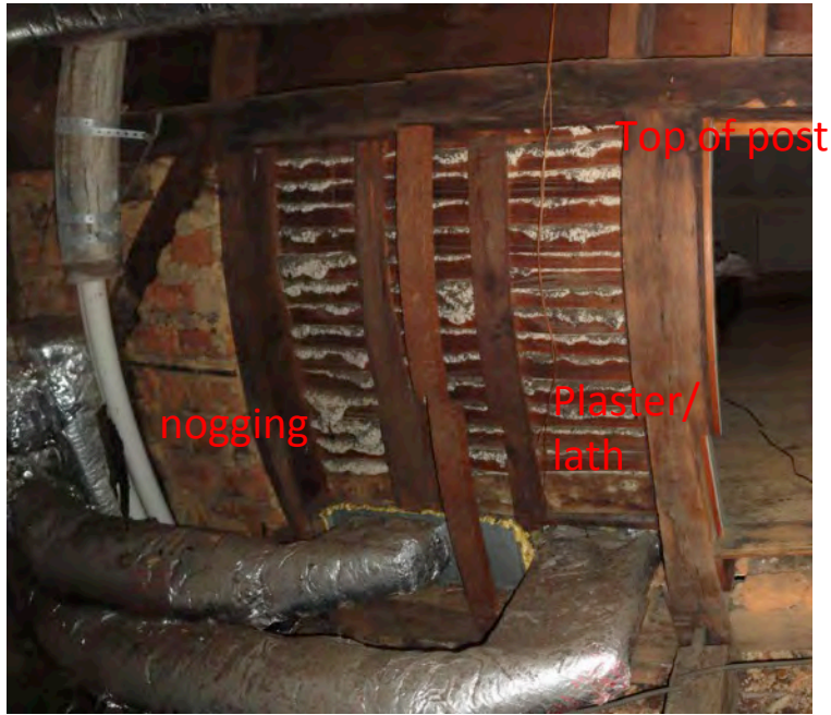
Above kitchen in Dutch House looking at original outside wall
