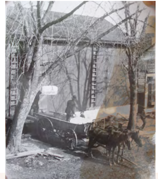
Loading ice blocks from 2 nd floor of barn into wagon
