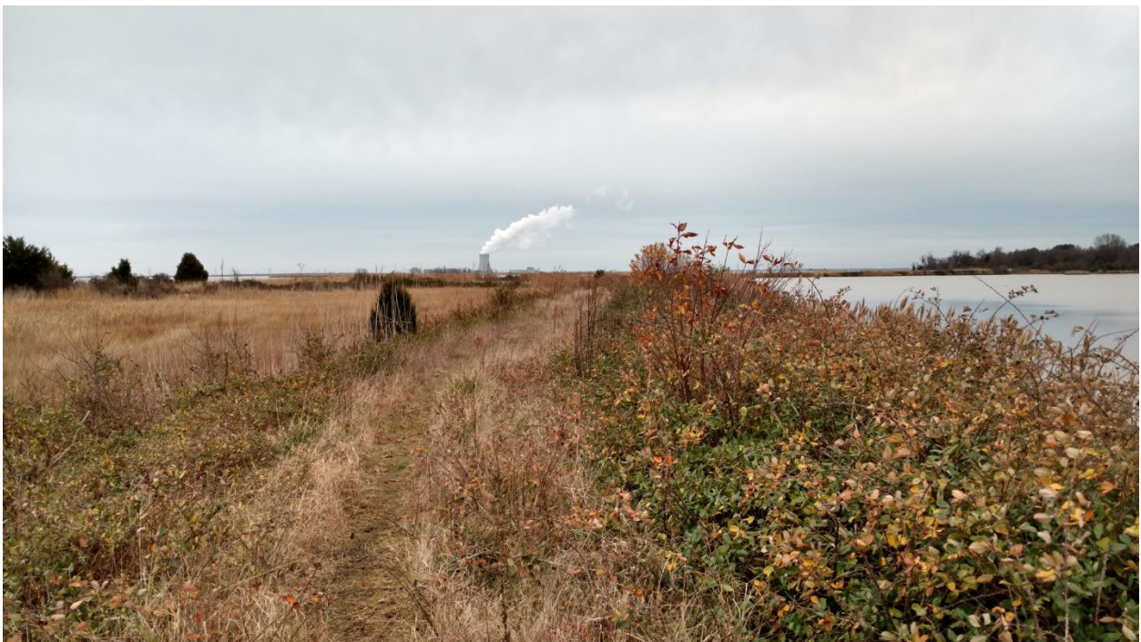
Figure 18. View to the south along the dog-leg portion of the embankment. The Lang Impoundment is to the right, and Salem I nuclear cooling tower is in the distance. Headquarters are in right background.
